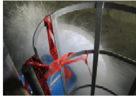
Fig.2: Back splash in the valve chamber.
