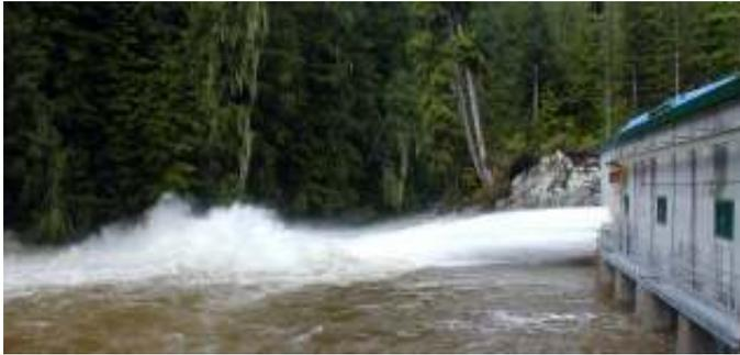
Fig.1: Valve discharge at 15% opening of the valve.
