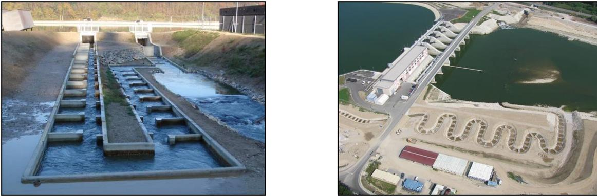
**Figure 1.** Fishway at HPP Arto – Blanca, Slovenia: the VSF reach (left), and the meandering reach.
